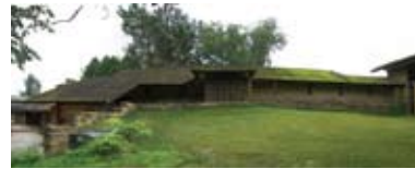
West Wing before restoration work.
