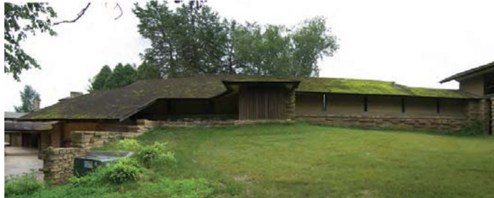
West Wing before restoration work.
