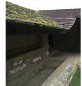
Ridge and framing condition above
