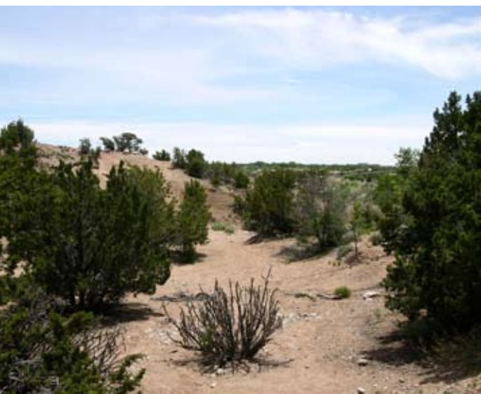
A: View from building site looking south
