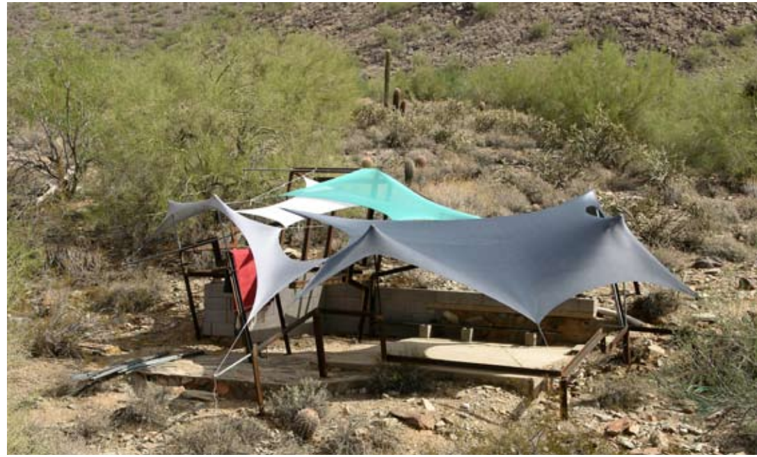
Full scale form finding process, using multiple pieces of spandex fabric
