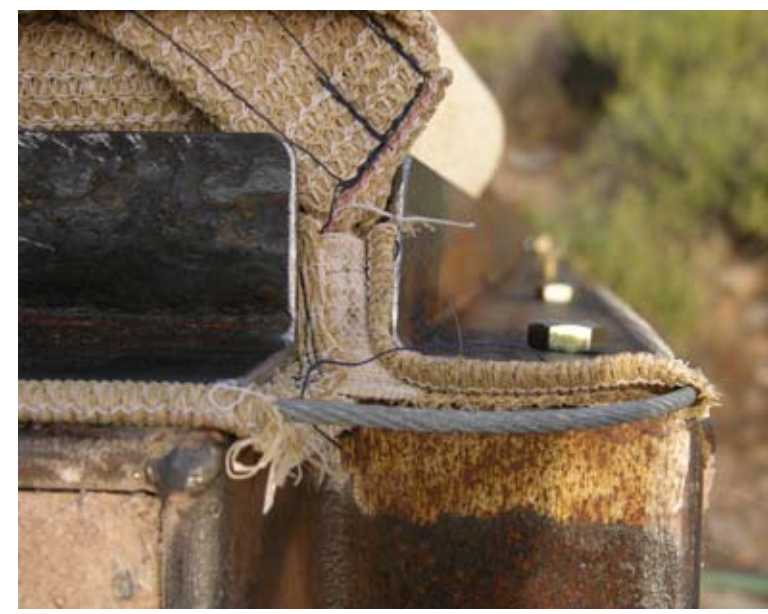
Mockup of fabric connection to the chimney mass
