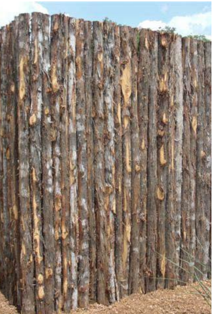
Commonly used as a fence material, Coyote Fencing was proposed to be applied horizontally as siding.
