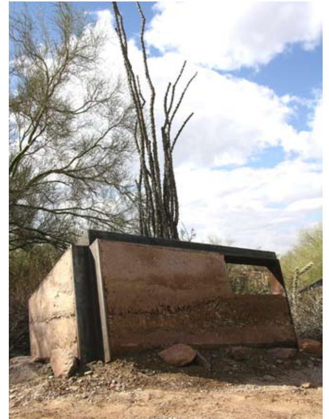
Completed mockup on site
