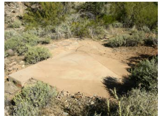
C: Existing hardscape looking to the northwest
