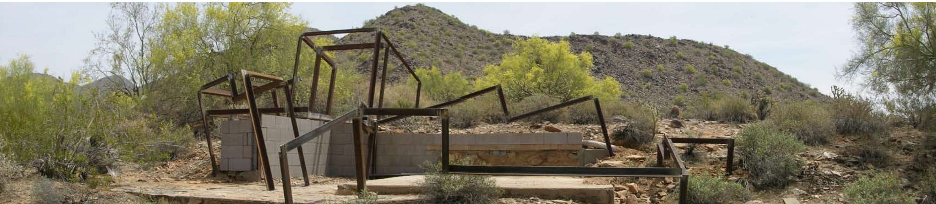
Rendering of the steel armature and 3" thick rammed-earth wall system
